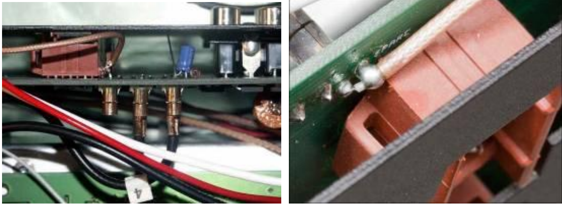
Figure A-4: Spare jack connection (Photo at right Courtesy of Roberto Barrios, EB4EQA)
